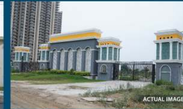
VICTORIAN VILLAS PLOTS & VILLAS RERA NO: UPRERAPR15838
